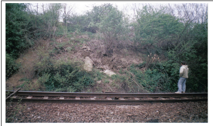
Figure 4. The land slip near the rail road
