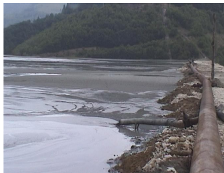
Fig. 3. – The decantation lake of Valea Şesei
